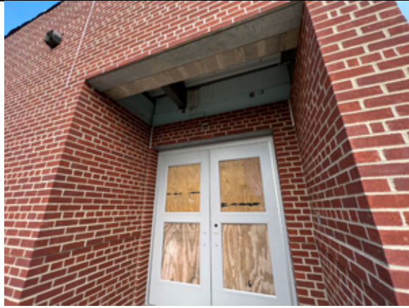
View of exit from the new addition onto the playground.
