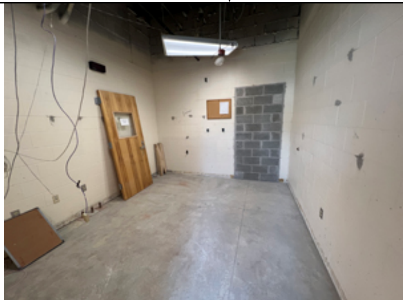
Opening have been infilled.
