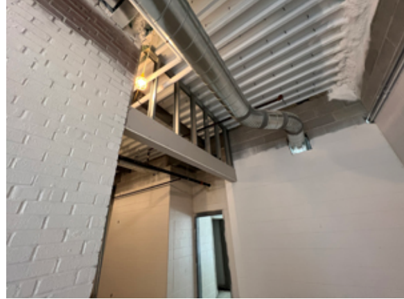
Work continues on the new addition.
