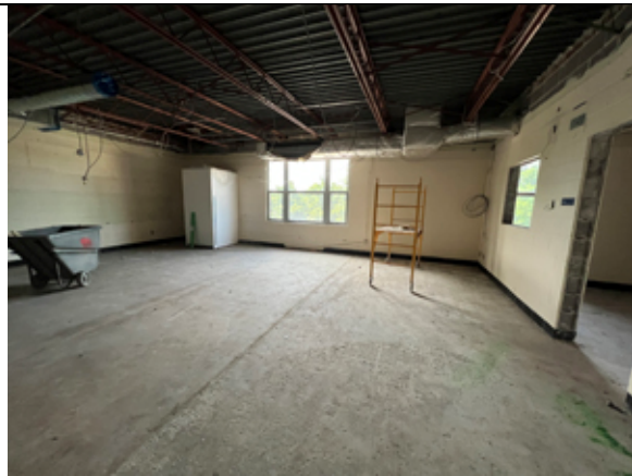
Demolition of the second floor is nearly complete.
