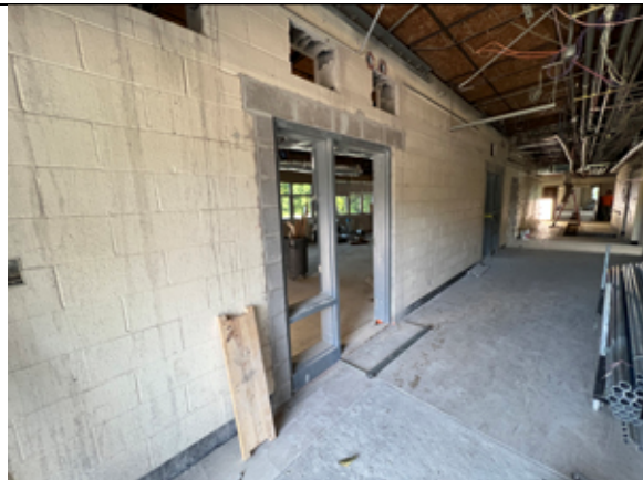
The new openings into the Admin Suite have been completed.
