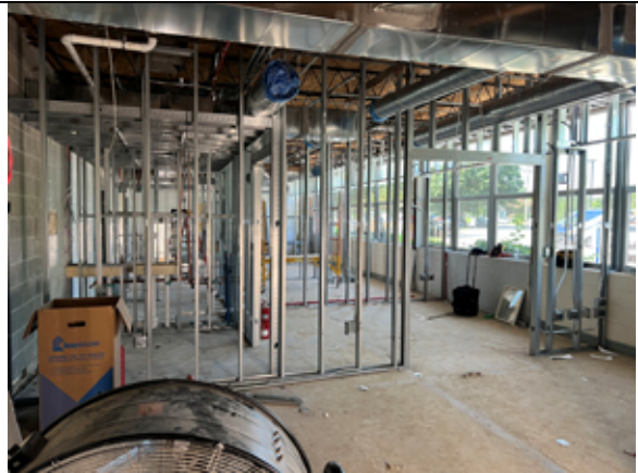
Framing and MEP rough-in's are nearly complete in the Admin Suite.
