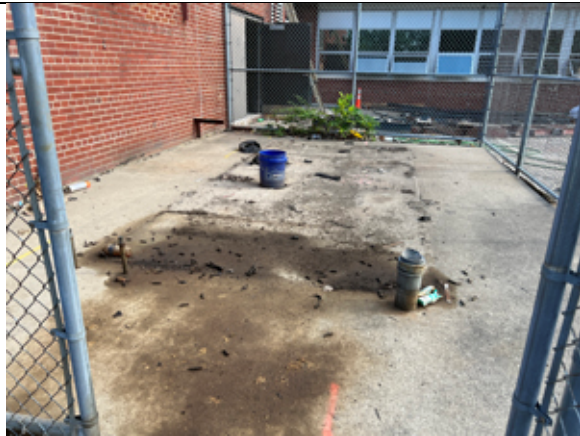
The old chiller has been removed.
