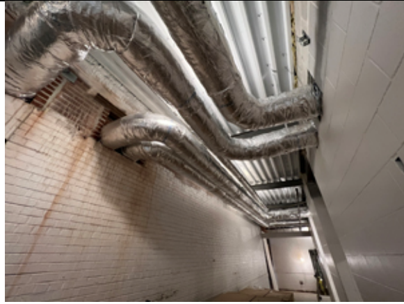
Ductwork is in the process of being insulated.
