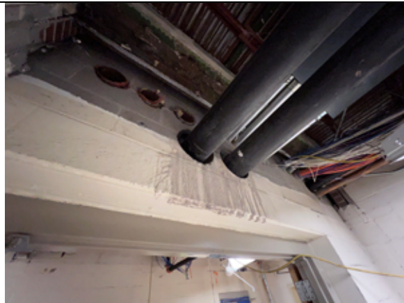
Existing and new MEP penetrations at the corridor wall between the original building and gym/media center addition have compromised the integrity of the bearing wall. The structural engineer will provide direction on how to reinforce the wall.
