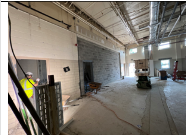
View of new wall between the Faculty lounge area and the Cafeteria.
