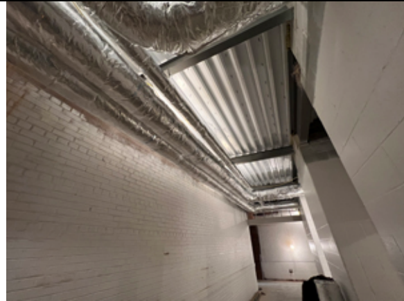
Ductwork is being insulated in the new addition.
