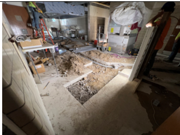
Installation of underslab utilities continue in the kitchen.
