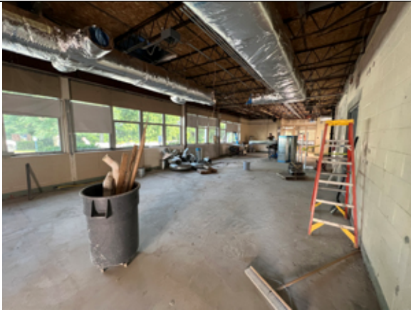
Installation of ductwork continues in the Admin Suite.
