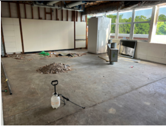
The original VCT has been removed from the second floor floors.
