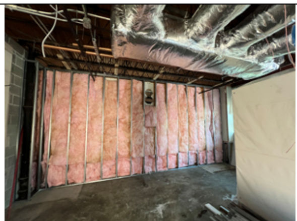
View of insulated wall between classrooms.
