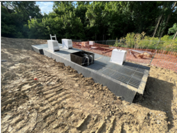
Installation of the new wastewater treatment plant is nearly complete
