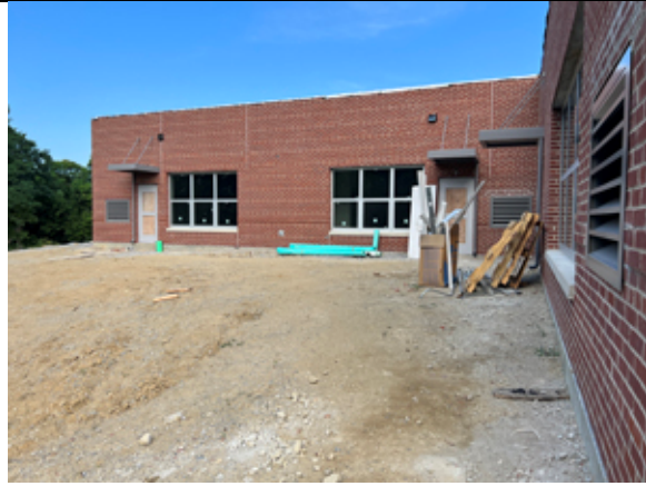
View of the area outside of the Pre-K classrooms.
