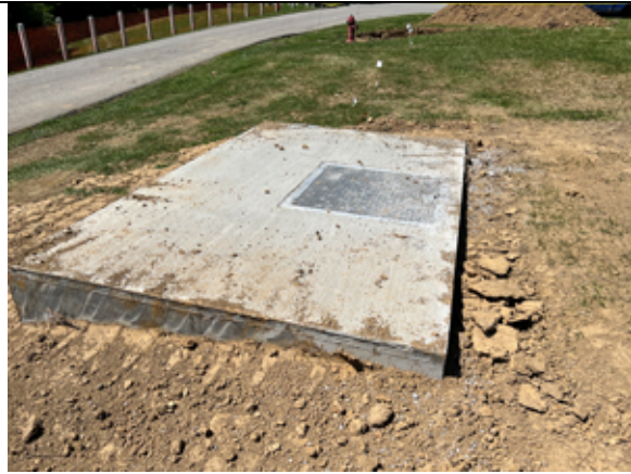
The new fire vault installation is complete.
