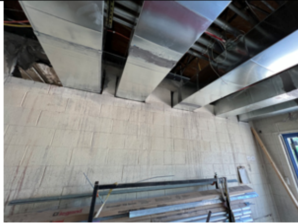
Installation of ductwork from the existing mechanical room.
