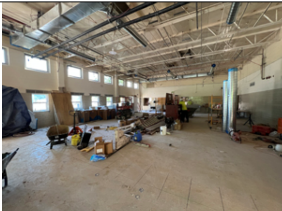
A view in the existing Cafeteria.
