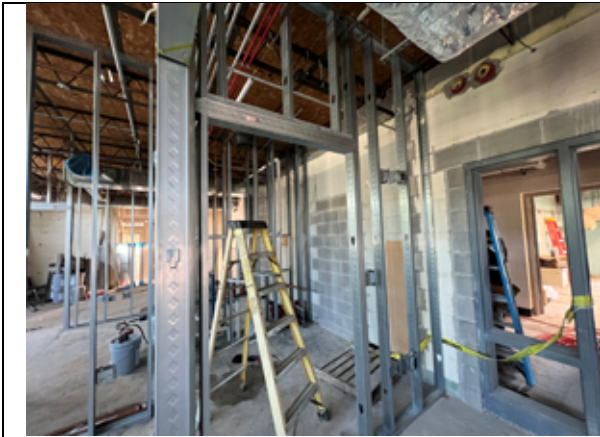
View of new stud framing in the Admin Suite.
