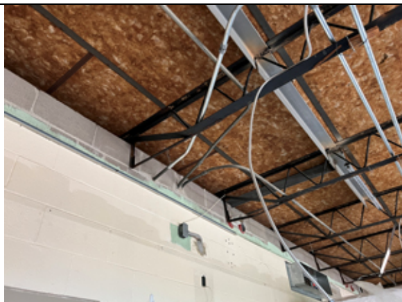
An existing masonry wall was compromised by previous MEP penetrations. These will be corrected per the structural engineers direction.
