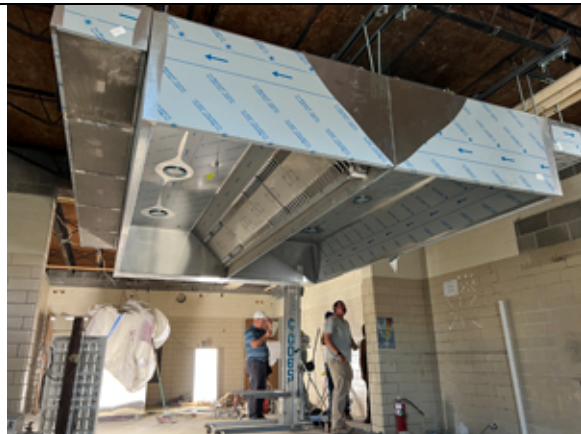
The new kitchen exhaust hood has been set.
