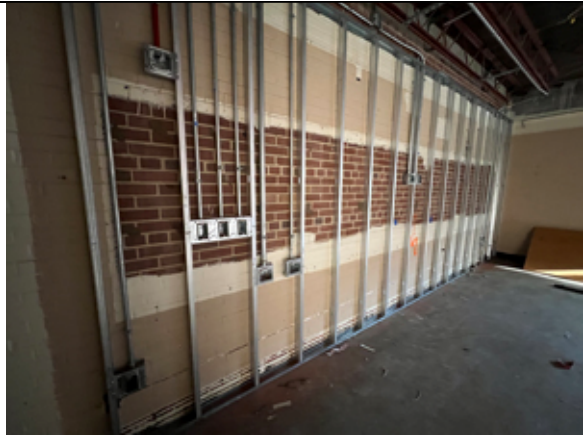
The classroom presentation wall framing and electrical rough-in has been completed.
