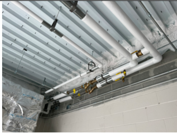
Piping is being insulated in the new addition.
