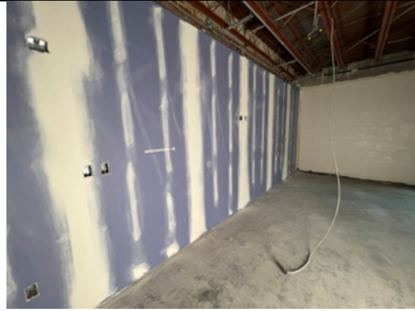
The presentation walls in the classrooms have been finished.
