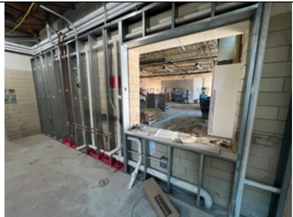
The new furred wall behind the dishwashing equipment.
