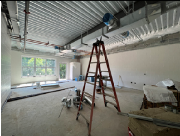
Work continues on the new addition.
