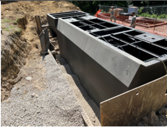
Installation of the new wastewater treatment plant is in progress.
