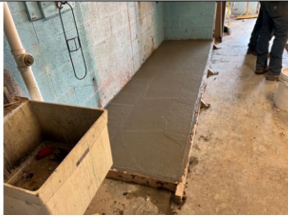
A housekeeping pad has been poured in the Mechanical Room.
