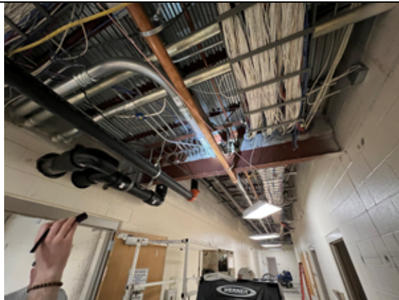
An existing masonry wall was compromised by previous MEP penetrations. These will be corrected per the structural engineers direction.
