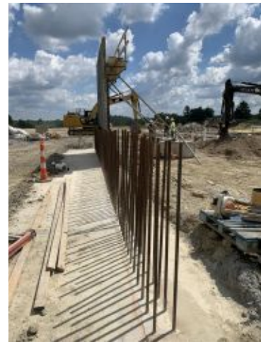
2022.07.13 – North wall of pool
