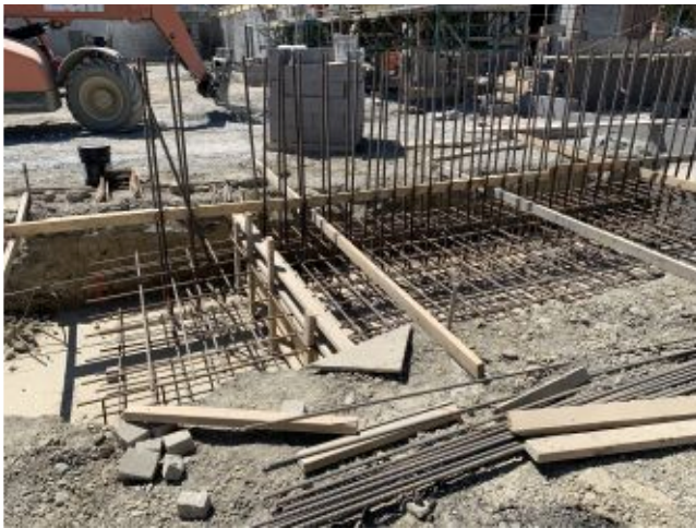
2022.06.30 – North wall of pool
