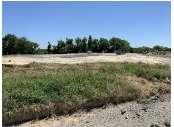
2022.06.30 – New tennis courts
