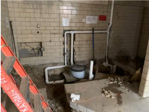
Ktichen under slab plumbing
