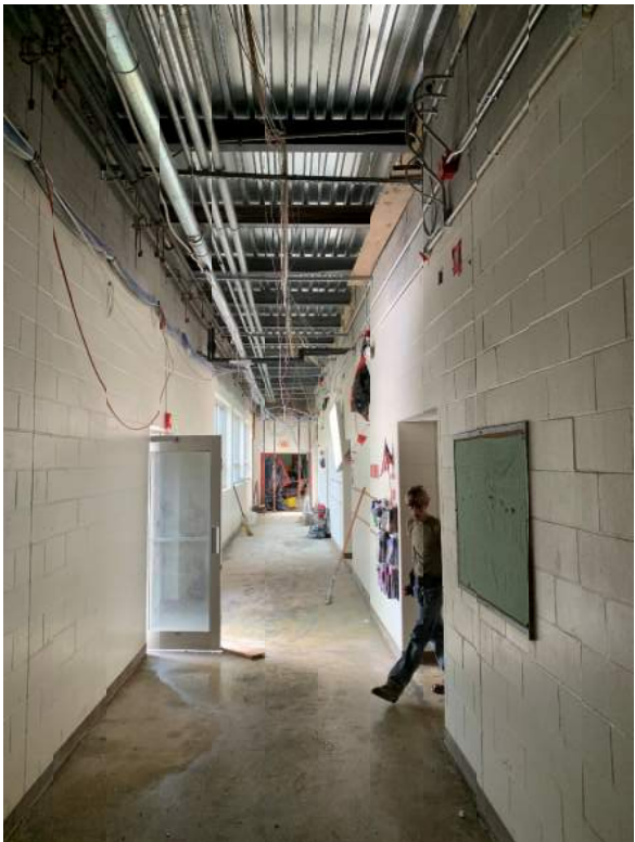
Classroom addition first floor corridor
