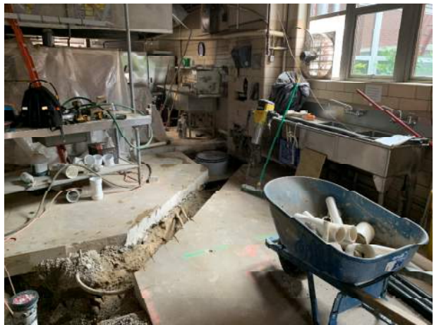
Kitchen under slab plumbing
