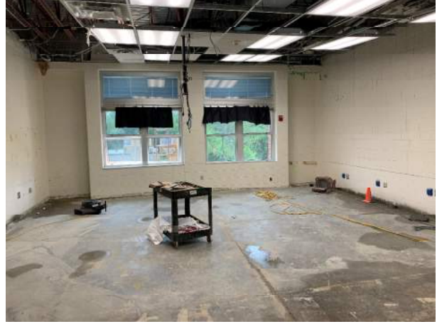
First floor classroom water damage demolition
