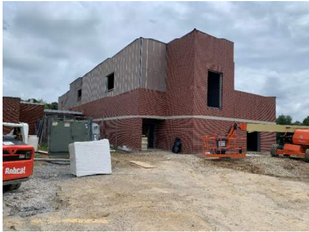
Classroom addition – west end, north elevation
