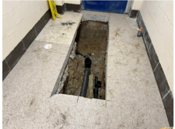
Repairs of the under-slab plumbing in the kitchen are in progress.
