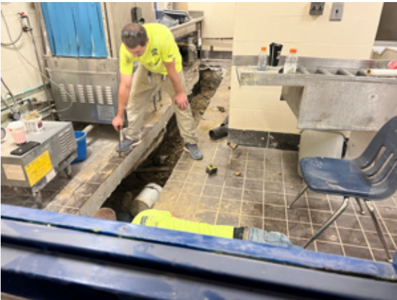
Repairs of the under-slab plumbing in the kitchen are in progress.
