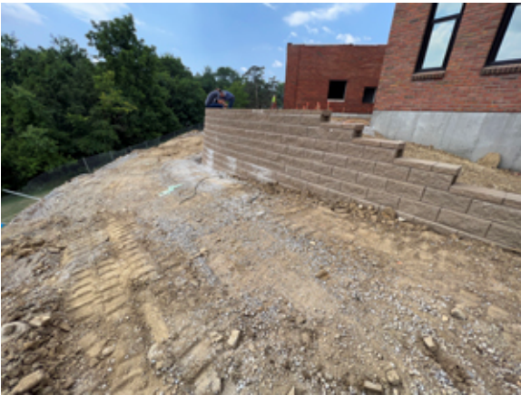
The new Allen Block retaining wall has been installed.
