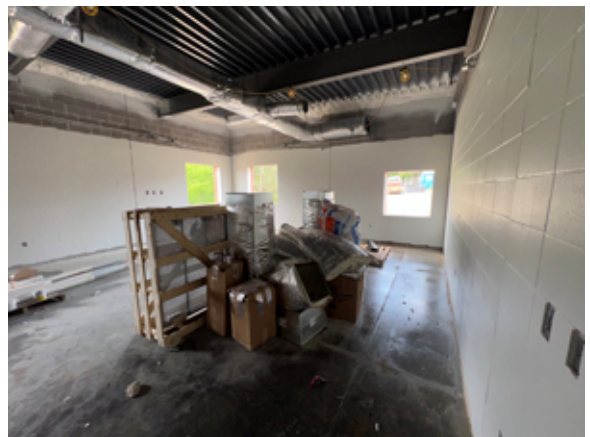
Ductwork has been insulated throughout.
