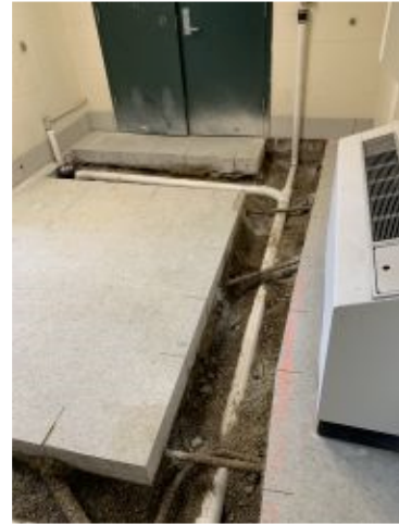
2022.06.23 - Below slab plumbing at Kitchen receiving
