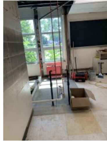
2022.06.23 – Plumbing at preschool restroom
