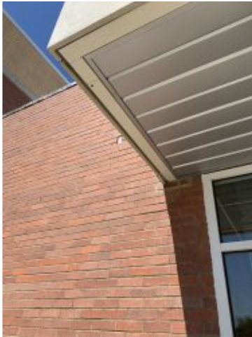
2022.06.23 – Installed soffit panels
