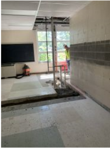
2022.06.23 – Plumbing at preschool restroom
