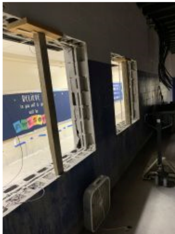
2022.06.23 – Window opening at former gymnasium
