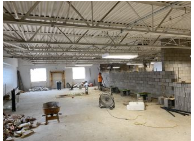
2022.07.07 – 2 nd floor classrooms
