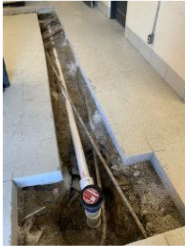
2022.06.23 – Below slab plumbing at Kitchen receiving
