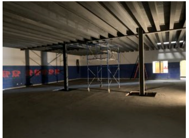
2022.06.23 – Floor infill framing at former gymnasium
