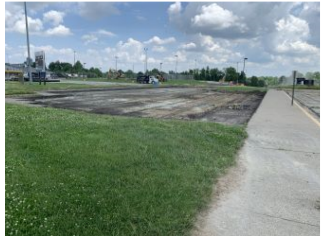
2022.06.01 – Milled asphalt at student parking
