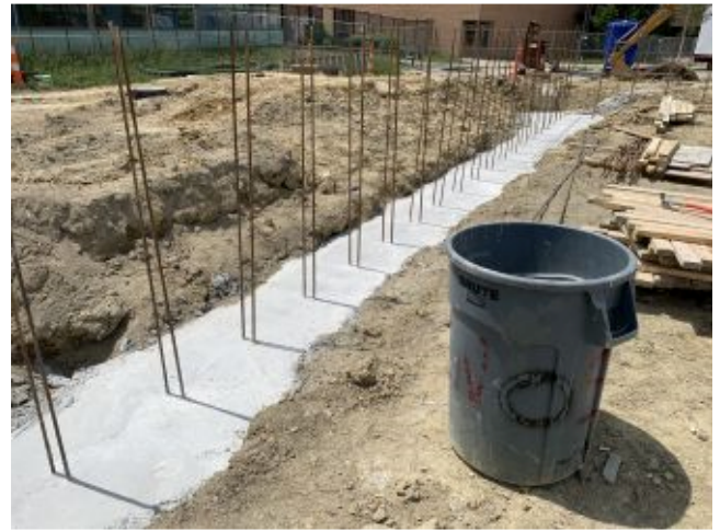
2022.06.01 – Grade beam at south wall of practice gym
