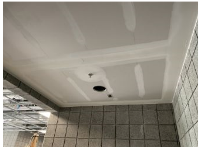
2022.06.09 – Drywall ceiling at restrooms
