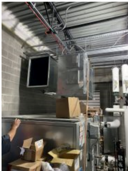
2022.05.26 – ERV at mechanical mezzanine
