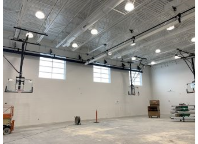
2022.05.26 – Backboards, divider, and archery net installed
