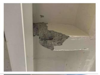
ITEM: 002-011 REMARKS: Paint all steel members. Paint should cover scrapes, welds, and slurry overflow from concrete pour.
