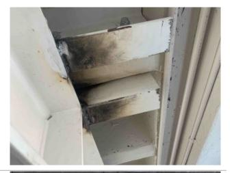
ITEM: 002-012 REMARKS: Concrete placed in holes from the upper levels. Finish is acceptable. This level and the bleachers need to be cleaned free of cement and dust.
