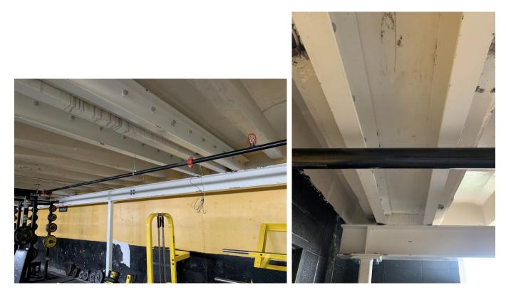
2. The gap between the channels and the existing concrete joists were within an acceptable limit.
