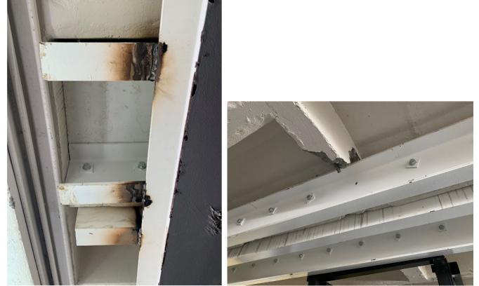
3. Refer to the photo on the left below. The channels have been welded to the supporting beam. It is not a structural concern, but the Architect should review the aesthetics of the welds.
