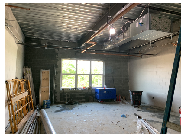
Typical new classroom – HVAC & electric r.i.
