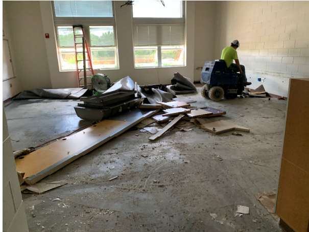
Existing first floor classroom flooring removal
