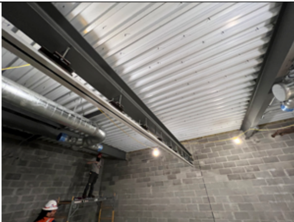
2022.05.31 The track for the folding partition has been installed.
