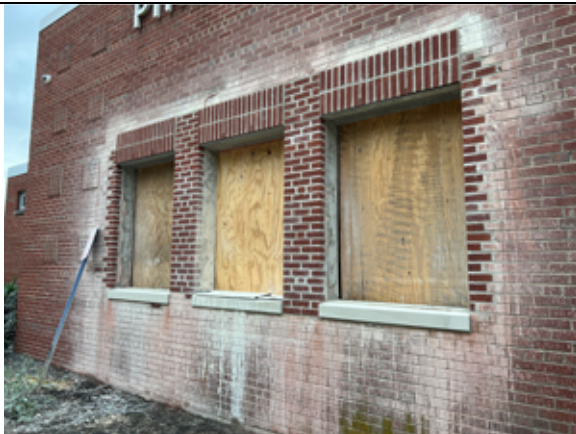
2022.06.14 Installation of the masonry openings at the new Faculty Lounge have been completed.
