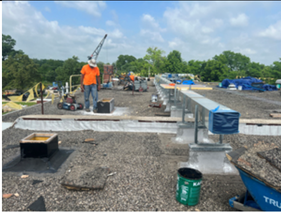
2022.06.14 Installation of equipment curbs continues on the existing roof.
