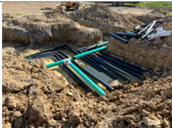
2022.05.31 Geothermal piping for the new mechanical room.
