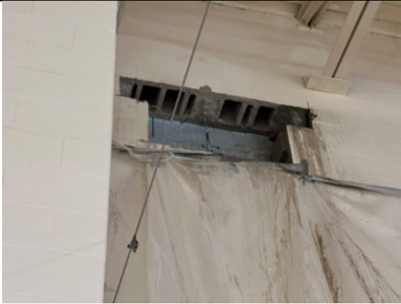
2022.05.31 New openings are being cut for the new ductwork in the gym.
