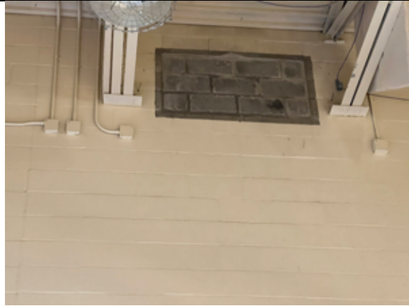
2022.05.31 Abandoned ductwork openings are being infilled.
