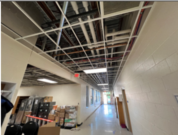
2022.05.31 Ceiling pads are being removed throughout the school.
