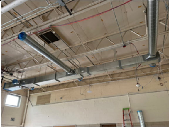
2022.06.07 Installation of HVAC ductwork continues with open ends being protected from dust.
