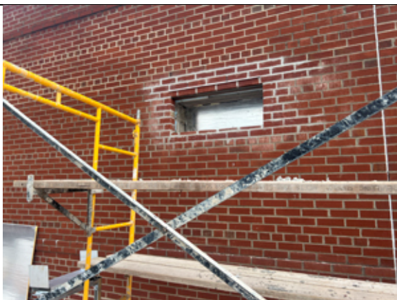
2022.06.14 Installation of the new HVAC louver opening in the gym.
