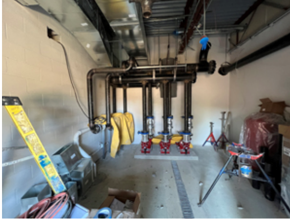
2022.05.31 Pumps for the new geothermal system have been installed.
