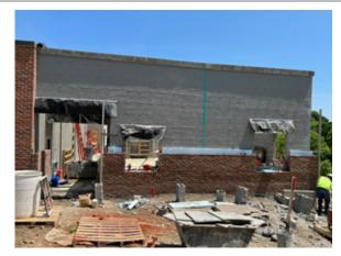
2022.05.24 Installation of the face brick has started.
