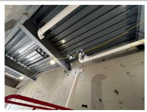
2022.06.07 Installation of the roof drains is in progress.
