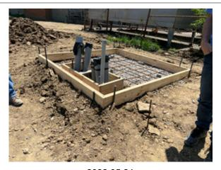
2022.05.24 Formwork for the new transformer pad.
