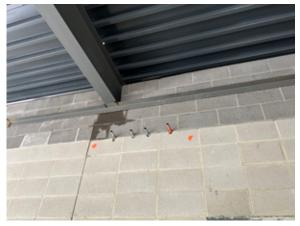
2022.06.07 Steel angle bracing for the top of masonry walls.
