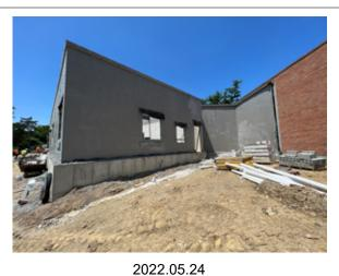
The air and water membrane has been installed over the exterior masonry.
