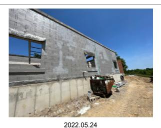
The air and water membrane has been installed over the exterior masonry.
