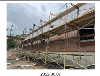
Installation of the face brick is in progress on the east elevation.
