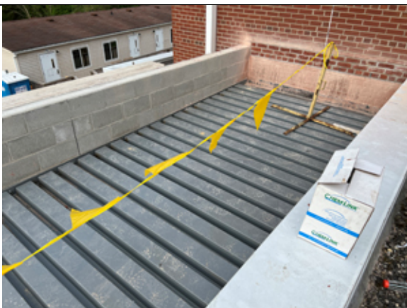
2022.04.26 Installation of the metal deck has been completed. Installation of the roofing and equipment supports has started.
