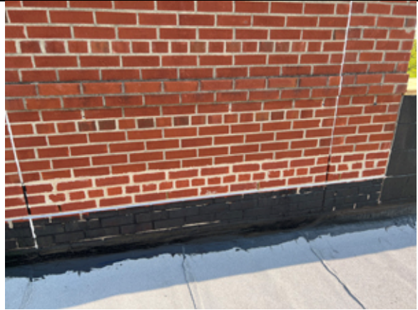
2022.05.10 The new counterflashing has been installed on the existing gym wall.
