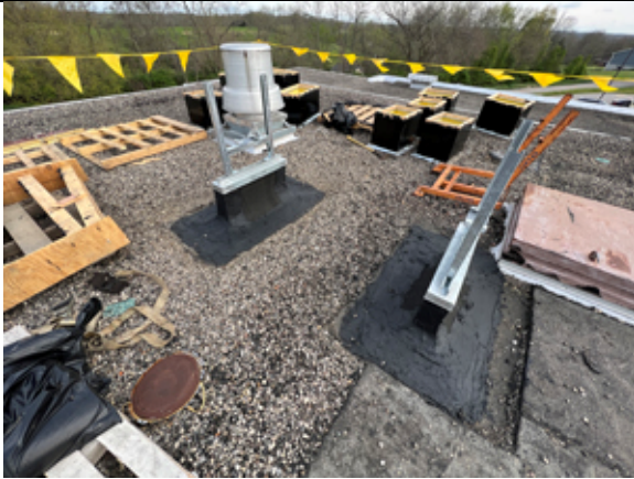
2022.04.26 Installation of the roof top equipment supports is in progress.
