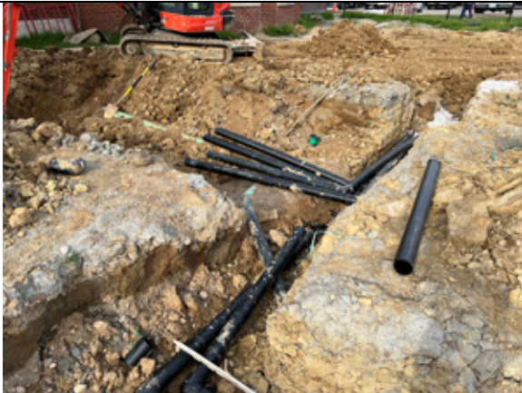
2022.04.26 The piping for the geothermal field is being brought into the building.
