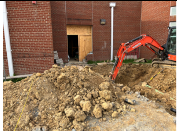
2022.04.26 The piping for the geothermal field is being brought into the building.
