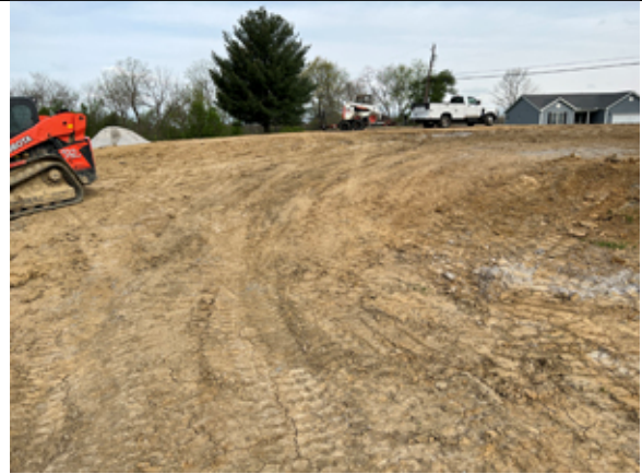
2022.04.26 The trenches for the geothermal field have been backfilled and graded.
