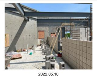
The installation of the steel roof framing is in progress. Installation of the ground-face concrete masonry is in progress.
