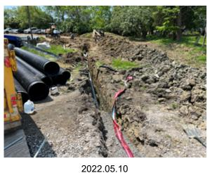
Installation of the new underground conduits for the electric service and fiber optic cable is in progress.
