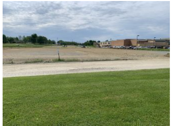
2022.05.18 – Final subgrade at fill parking
