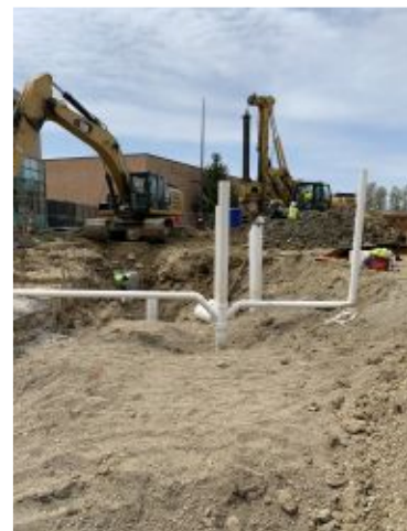
2022.04.29 – Installing sanitary/storm and pier
