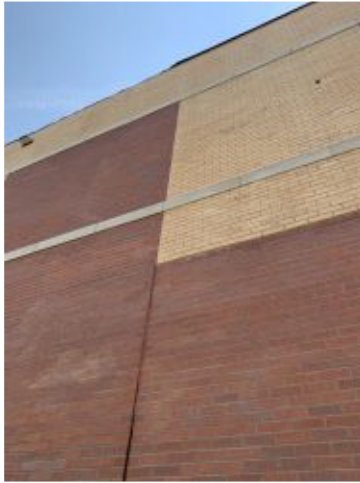
2022.05.12 – Partial control joint installation
