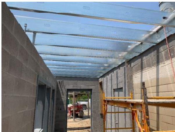
Kitchen addition roof framing
