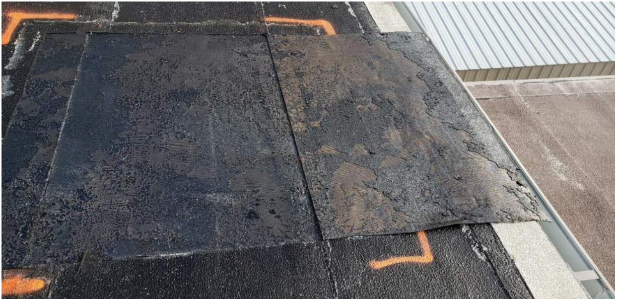
Photo 8: T-1 – Mode of Failure noted between cap sheet and inter-ply membranes, poor adhesion as evidenced by discolored areas of the roof membranes affected by moisture.
