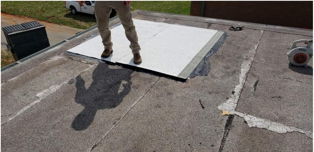
Photo 12: Repairs by Swift Roofing. Completed 1-ply granule surfaced modified bitumen cap sheet set in cold process adhesive.
