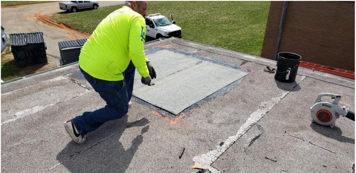
Photo 10: Repairs by Swift Roofing. Completed 1-ply smooth surfaced modified bitumen roof membrane set in cold process adhesive.
