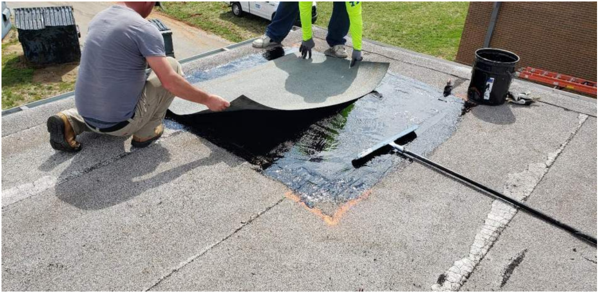
Photo 9: Repairs by Swift Roofing. 1-ply smooth surfaced modified bitumen roof membrane set in cold process adhesive.
