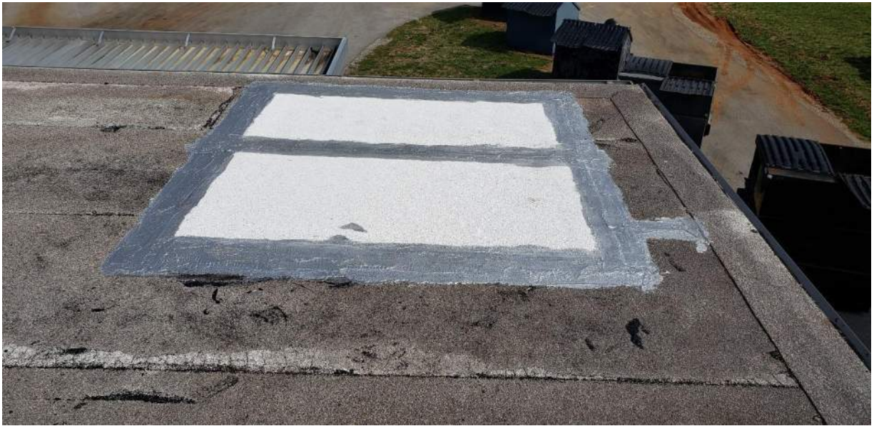
Photo 13: Repairs by Swift Roofing. Finished repair with all laps sealed with a 5-courses of membrane and mastic.
