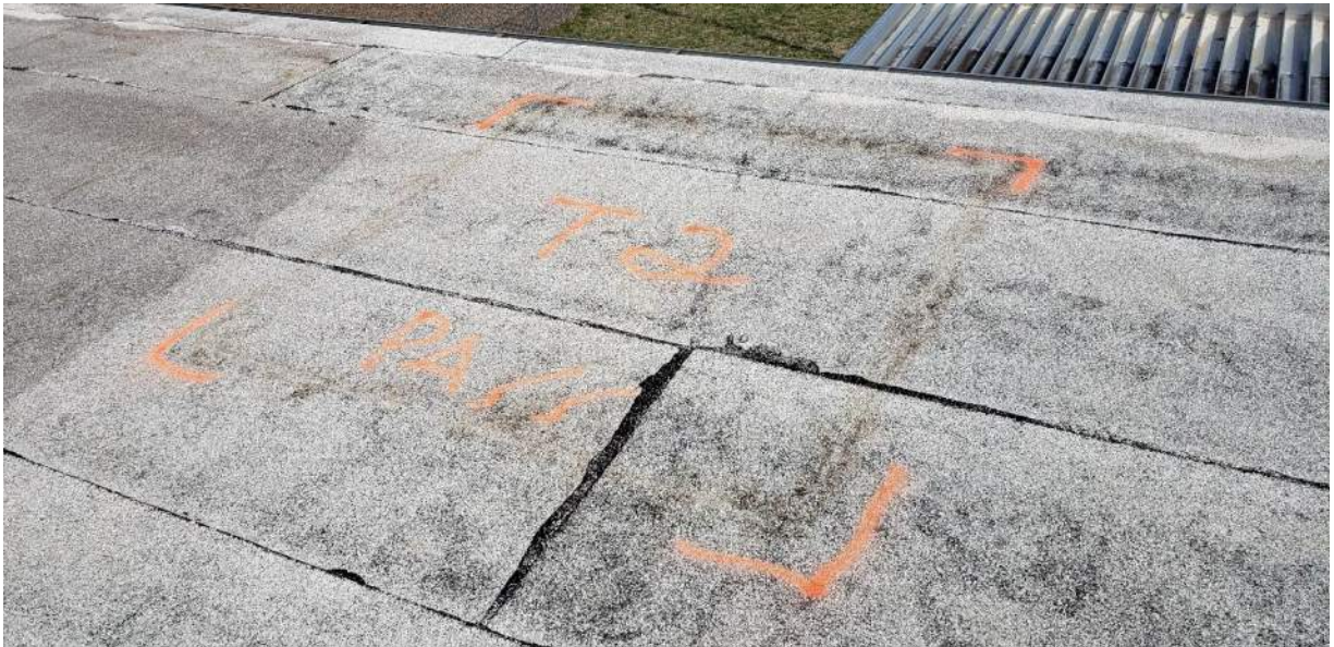
Photo 2: Typical test area, marked and numbered.
