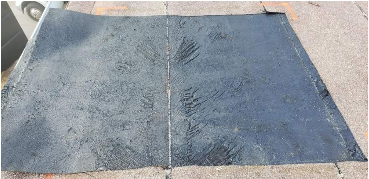
Photo 4: T-1 – Mode of Failure noted between cap sheet and inter-ply membranes, poor adhesion as evidenced by smooth separation of the roof membranes.
