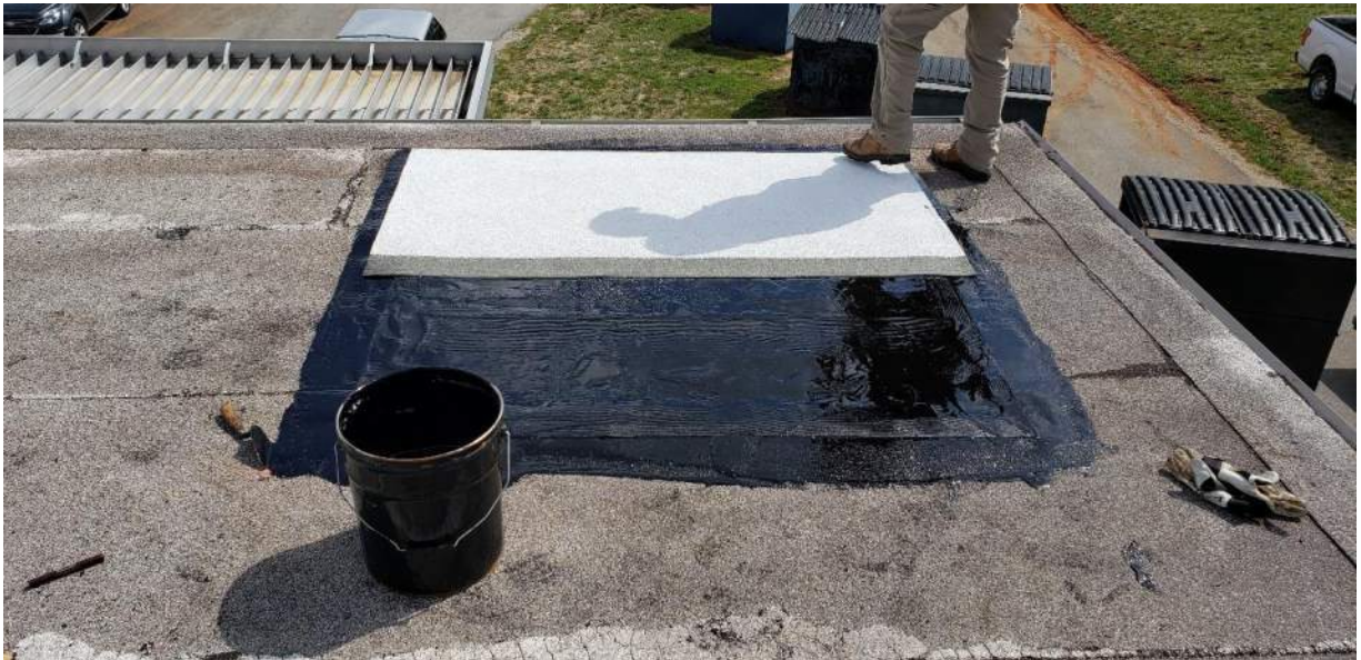
Photo 11: Repairs by Swift Roofing. 1-ply granule surfaced modified bitumen cap sheet set in cold process adhesive.
