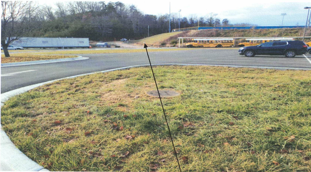
Picture of unknown Manhole #2, the questionable unknown pipe is from manhole to the sign seen in the distance, line representing the expectant routing of 4" PVC sewer pipe.
