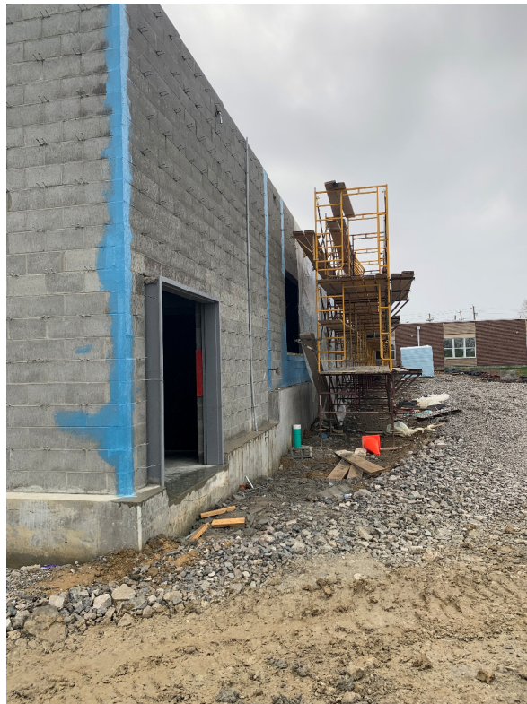
West elevation – moisture barrier installation
