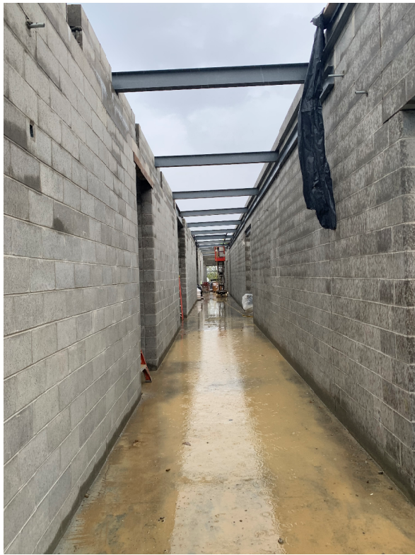
North-south corridor roof framing
