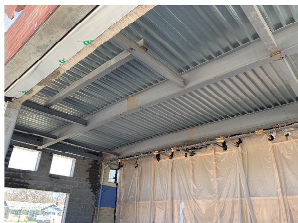
Cafeteria addition – roof framing
