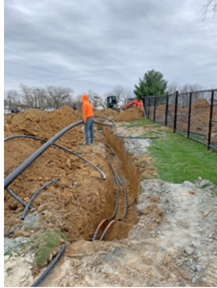
2022.03.29 Installation of the geothermal well field continues.
