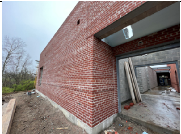
2022.04.12 Installation of the face brick continues.
