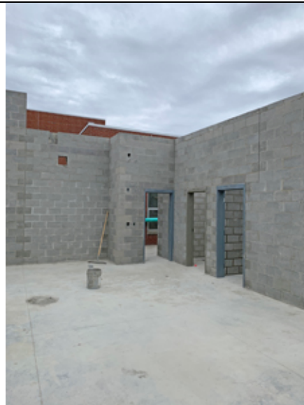
2022.03.29 Interior masonry walls.
