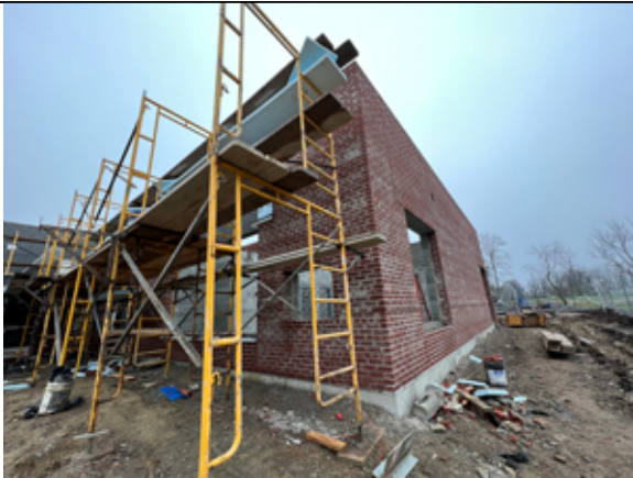
2022.04.12 Installation of the face brick continues.
