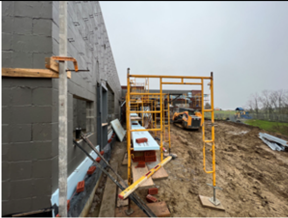
2022.04.12 Installation of the face brick continues.
