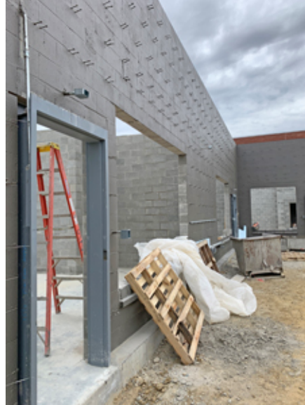
2022.03.29 Installation of the air and water membrane on the masonry walls is in progress.
