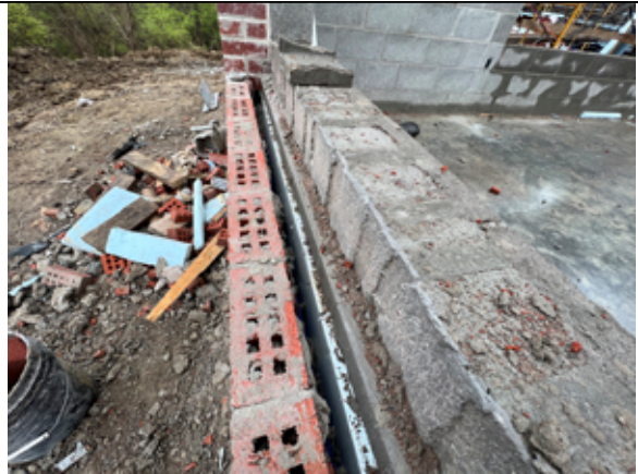
2022.04.12 Installation of the face brick continues.
