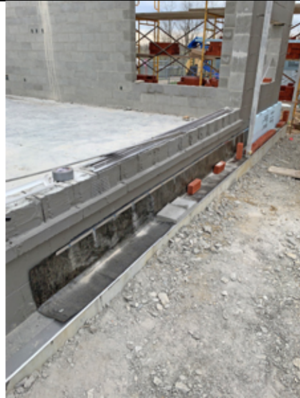
2022.03.29 The thru-wall flashing and stainless steel drip edge are being installed.
