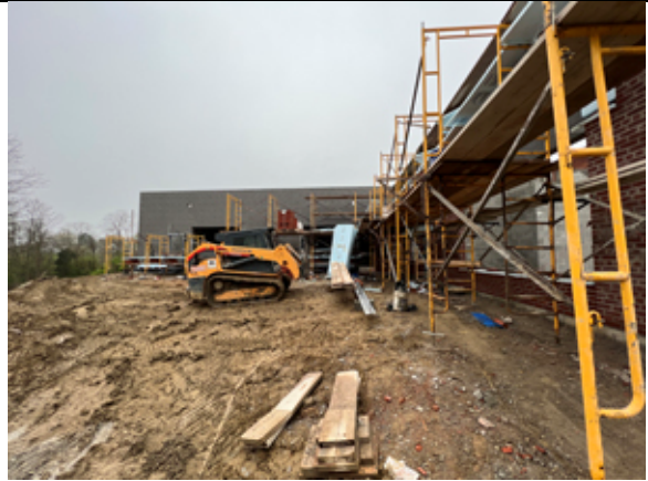
2022.04.12 Installation of the face brick continues.
