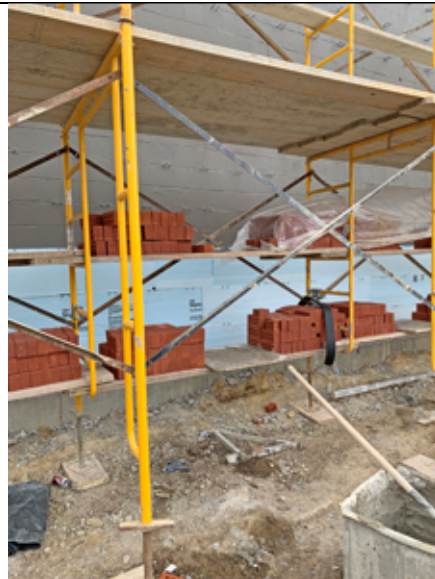
2022.03.29 Installation of the exterior brick and backup rigid insulation has started.
