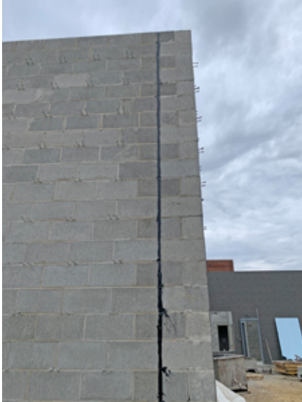
2022.03.29 The control joints in the exterior masonry walls are being caulked.
