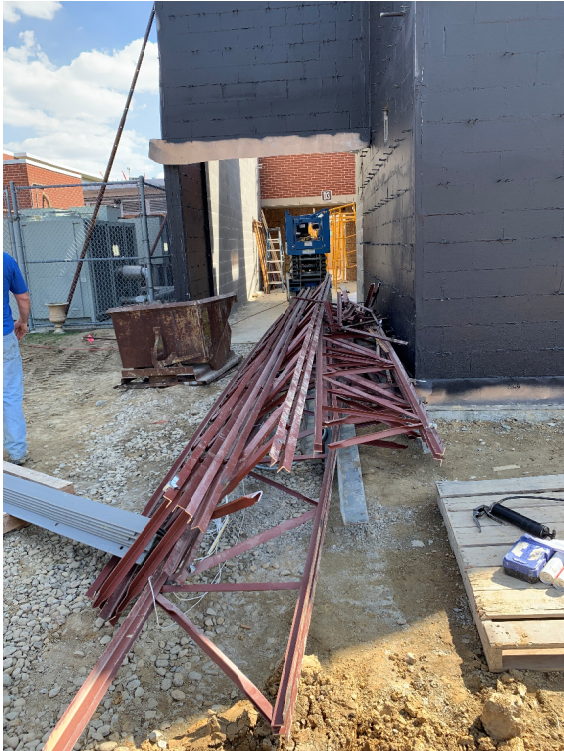
Classroom wing addition – removed roof joists
