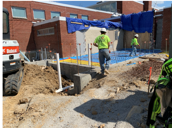
Kitchen addition foundation and slab prep
