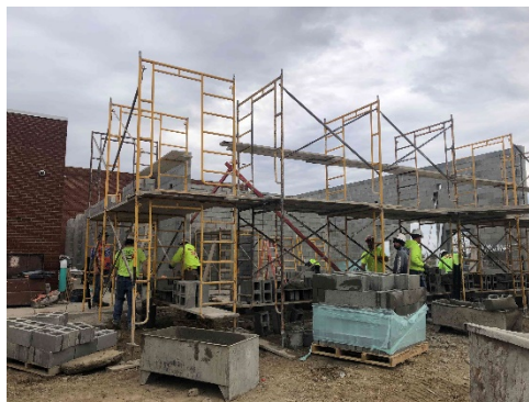
2022.03.15 CMU bearing walls are in progress.
