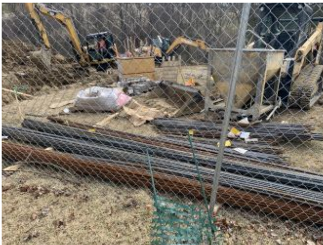
2022.03.01 – Rebar staged for use in footings.
