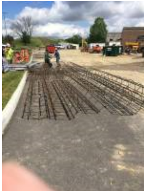
2017.06.15 – rebar cages for Phase 2 piers
