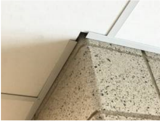
2017.06.15 – missing preformed grid corner
