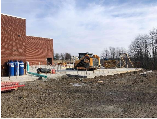
2022.02.01 The new door frames are being set.
