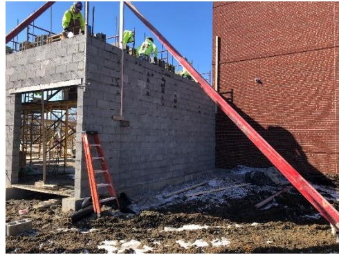
2022.02.15 CMU bearing walls are in progress.
