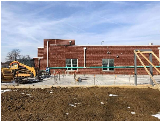
2022.02.01 The new door frames are being set.
