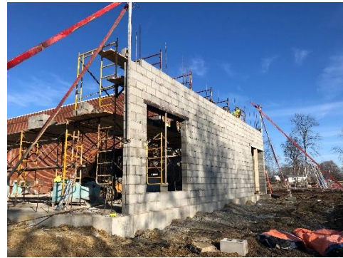
2022.02.15 CMU bearing walls are in progress.
