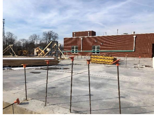
2022.02.01 The new door frames are being set.
