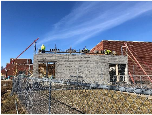
2022.02.15 CMU bearing walls are in progress.
