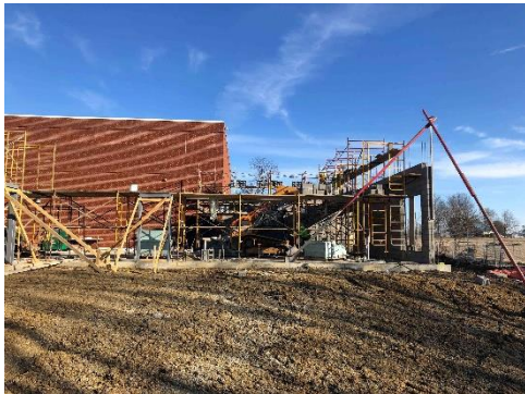
2022.02.15 CMU bearing walls are in progress.
