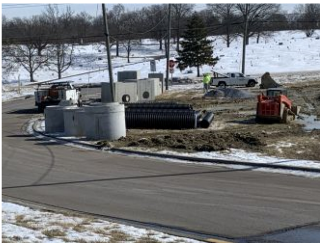
2022.02.09 – Storm structures staged for installation.
