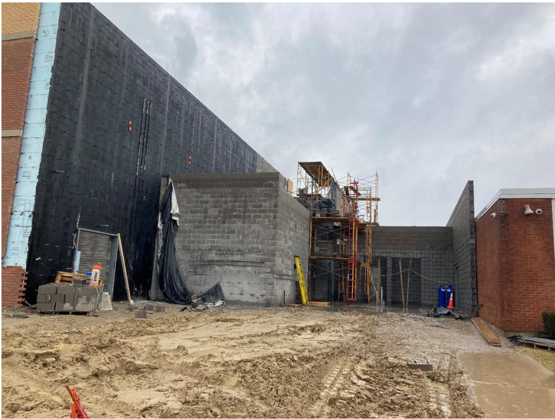
Masonry for mezzanine along with mezzanine door going up
