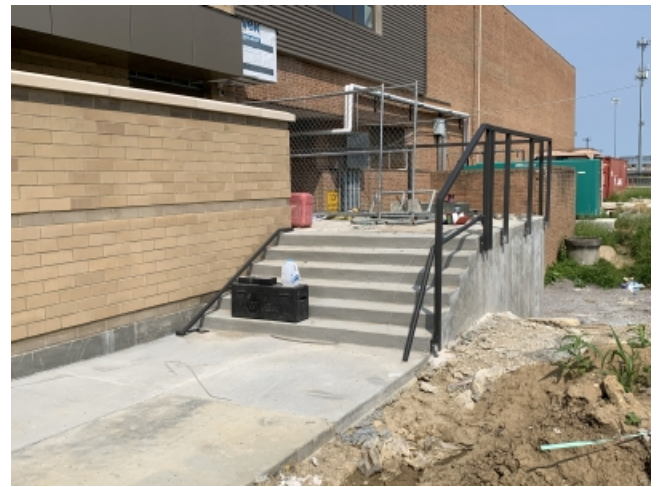
2019.06.05 – Guard rail installation
