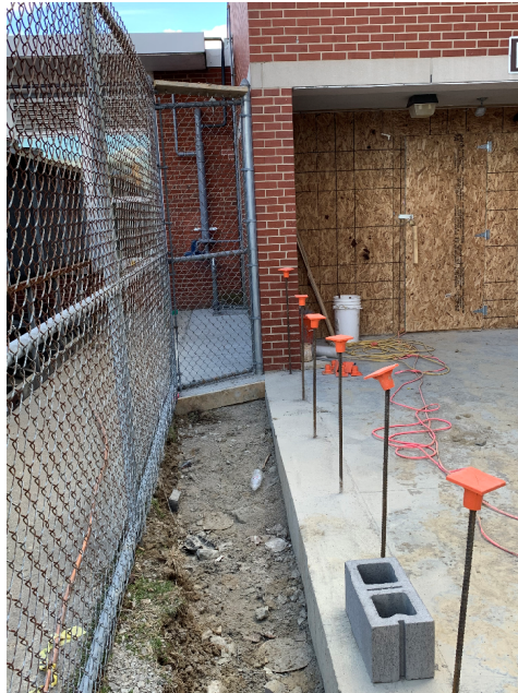
New gas piping at building
