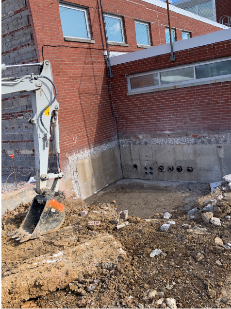
Demolished former electrical vault
