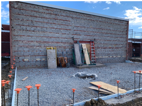
Cafeteria addition – completed foundations & slab prep. Wall demolition started
