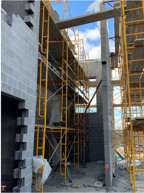
Interior view of new stairwell
