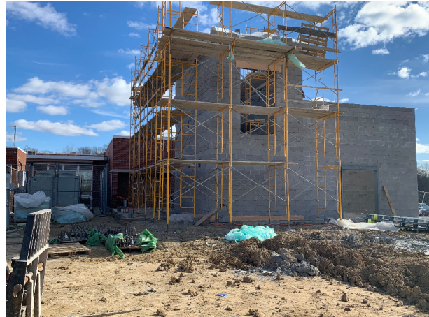
Stair/elevator addition exterior cmu walls
