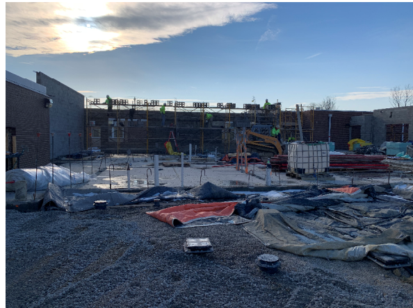
South/east walls of addition – Preschool classrooms
