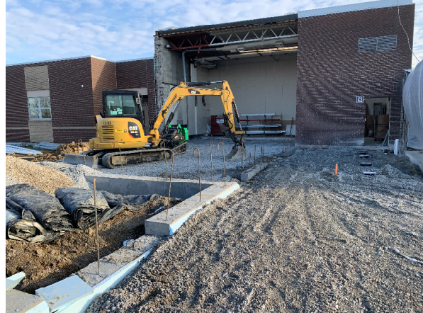
Slab prep at kitchen and cafeteria addition
