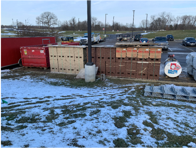
Brick veneer on site
