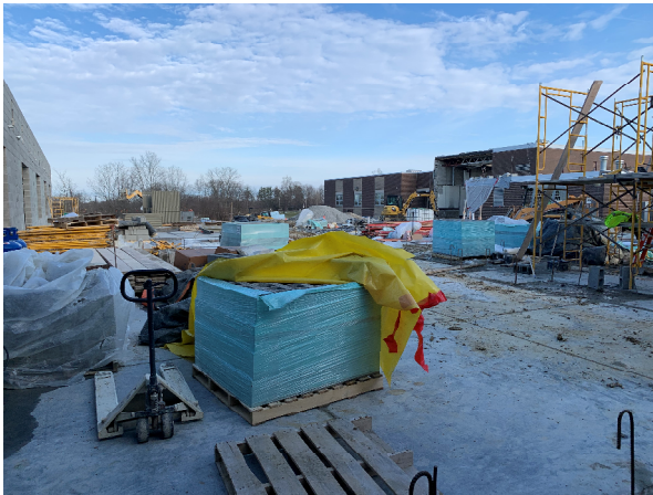
View from southwest corner of addition looking North
