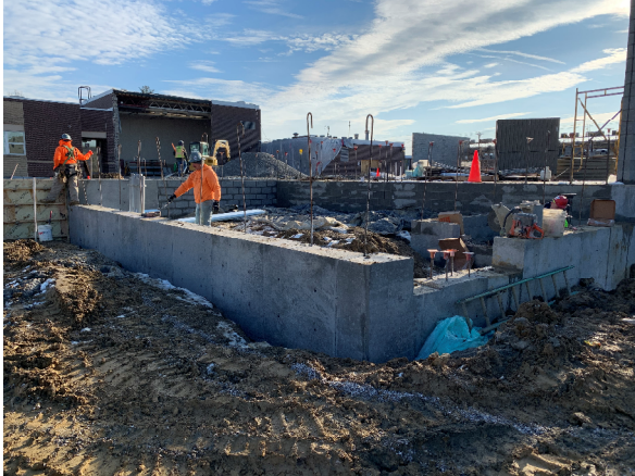
Northwest corner of addition – storage room
