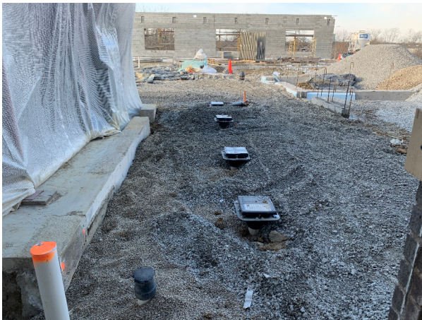
Kitchen floor drains – West exterior wall beyond
