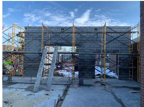
Southeast wall looking into Preschool courtyard
