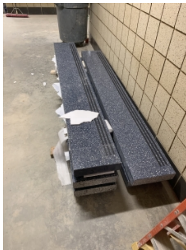
2019.05.07 – Precast terrazzo staged for installation
