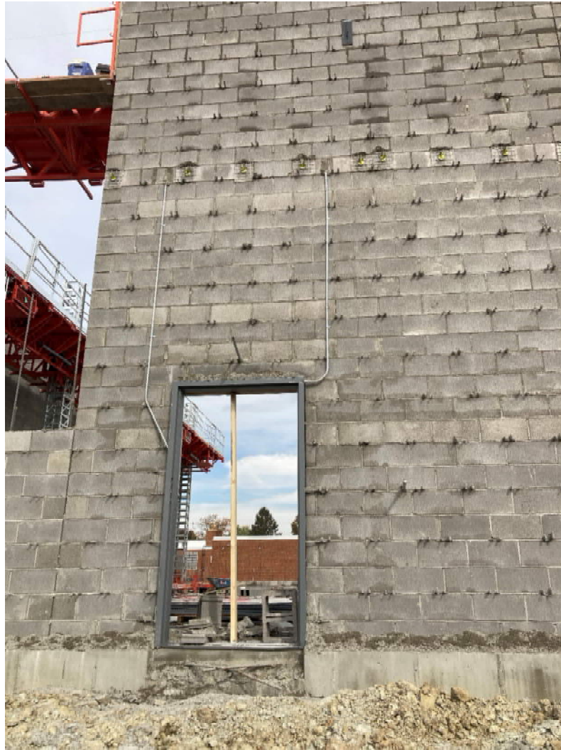
Door installed in CMU. (Electrical rough-ins and masonry anchorage visible)
