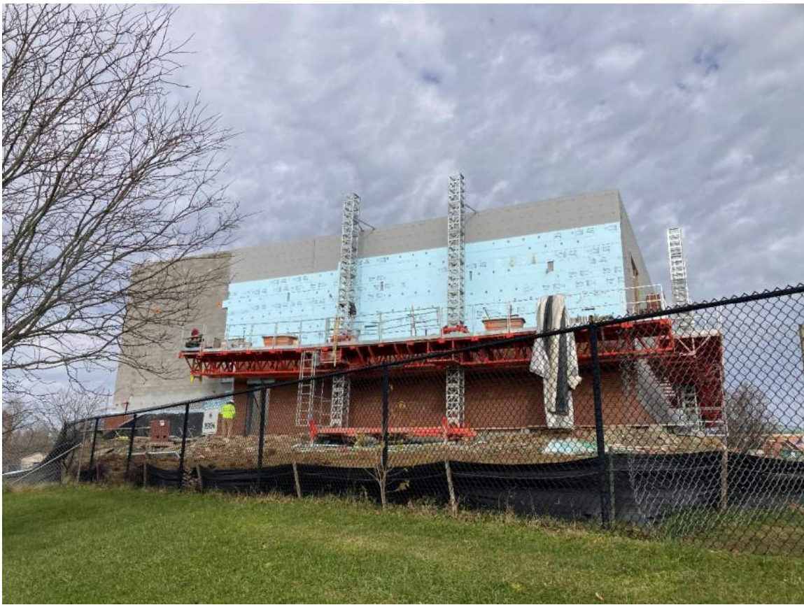
Southern face of gymnasium (spray-applied air barrier, insulation, and brick all visible)
