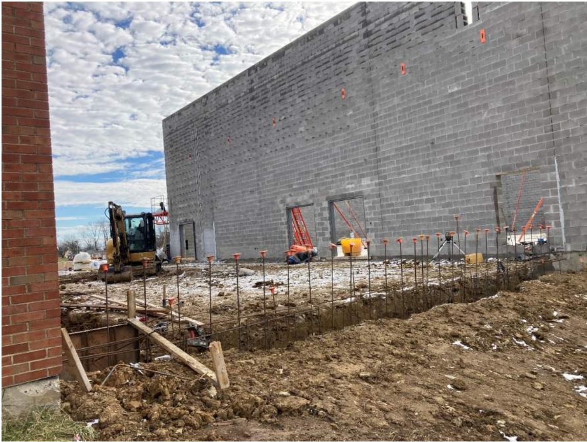
Footings cut and prepared for concrete pour
