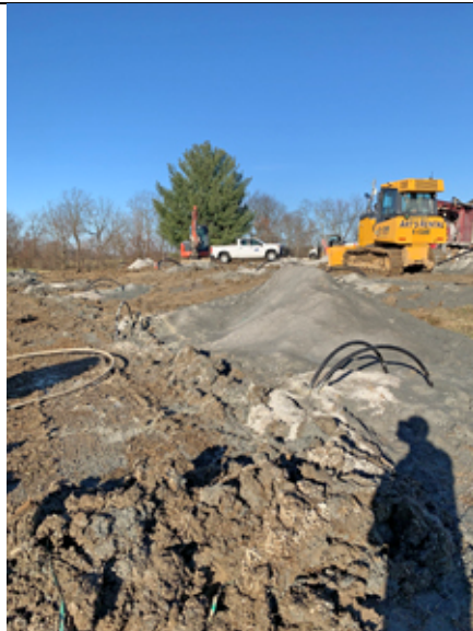
Installation of the geothermal well field continues.
