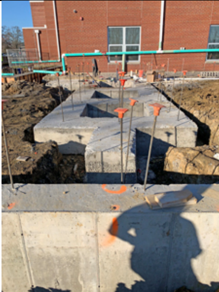
Installation of the perimeter grade beams and foundations walls appears to be complete.
