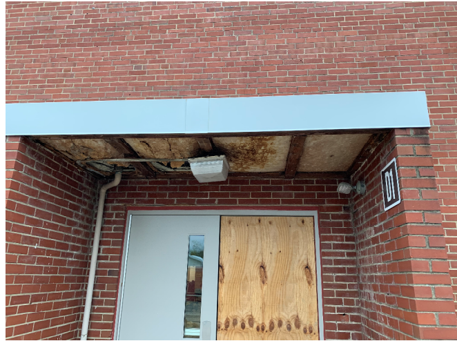
Asbestos soffit panels removed – cafeteria canopy
