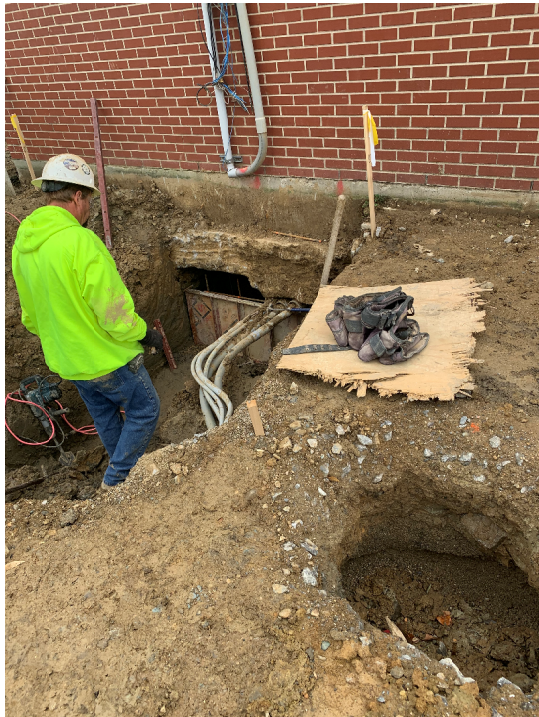
Foundation underpinning at future elevator
