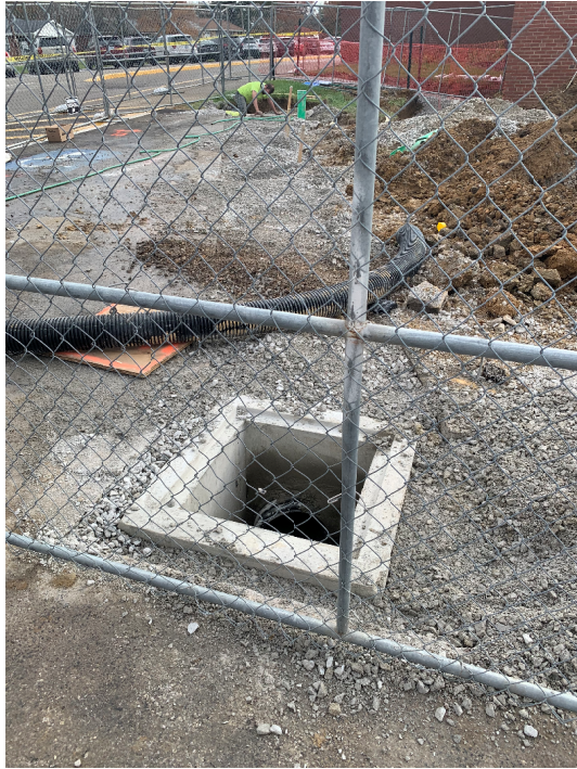
Catch basins and piping at north side of cafeteria addition
