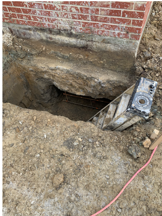
Foundation underpinning at future elevator
