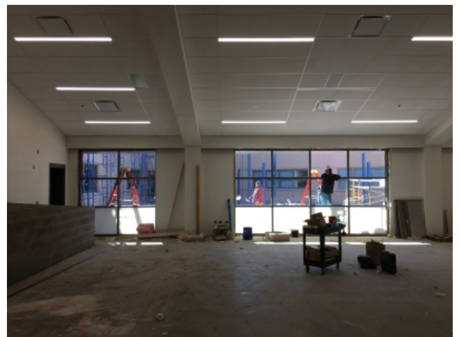
2019.03.26 – Installing storefront glazing
