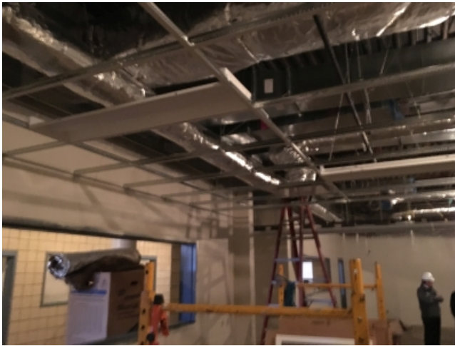
2019.02.12 – Light fixture in grid at upper level.
