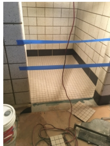
2019.02.12 – Installed floor tile.
