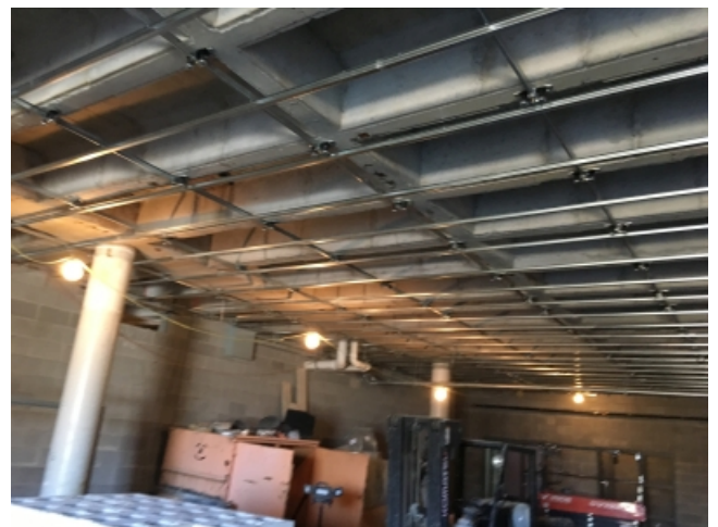
2018.12.18 – Band room sound isolating ceiling framing.
