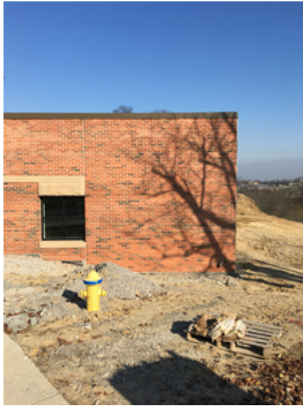
2018.12.10 – The roof coping has been installed.
