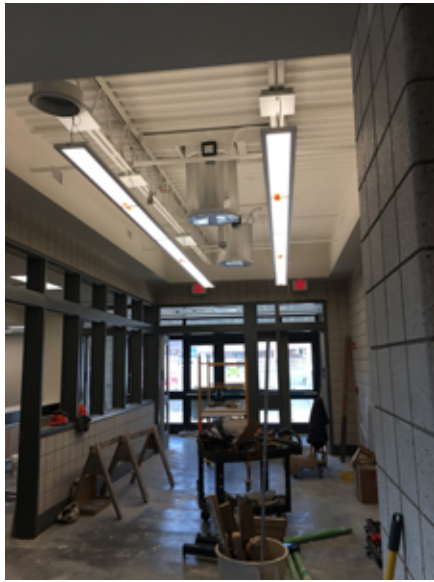
2018.12.10 – Light fixtures have been installed in the Lobby.
