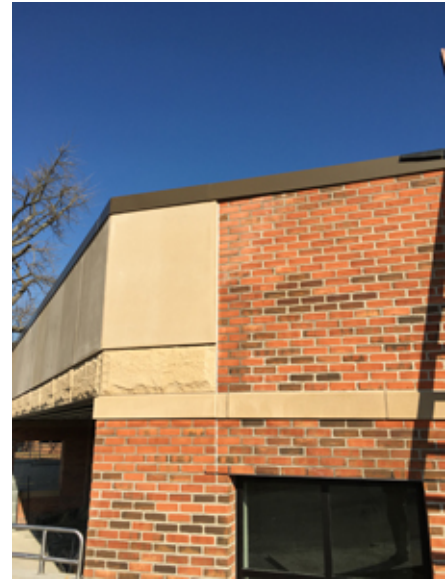
2018.12.10 – The roof coping has been installed.
