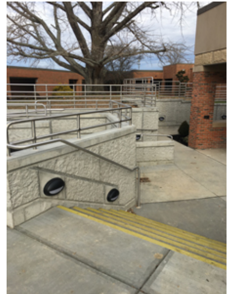
2019.01.07 – The exterior concrete stairs have been repoured.
