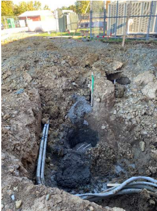
STAIR-ELEVATOR ADDITION Drilled piers/rerouted electric service Temporary propane tanks in background
