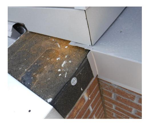
f) The joint between the brick pier and the structural steel canopy support has a mortar joint. As temperature change the steel will expand at a different rate than the masonry. The mortar must be removed in the joint between the steel and masonry and a soft sealant joint installed.
