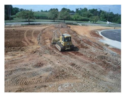
d) The area between the classroom wings has been rough graded after the storm piping was installed. The landscaper must apply the topsoil and the lawns in these areas.
