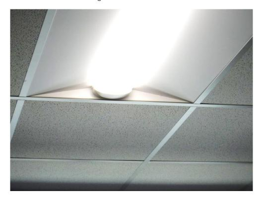
x) Ceiling grid must be straight, and the tiles must be fully seated in the grids.
