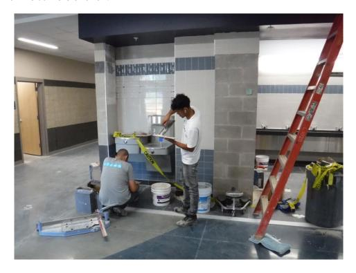
r) The PR included raising the height of the blue tile above the wash station to match the raised blue band on the corridor walls. The blue band must be raised as indicated on the PR drawing.
