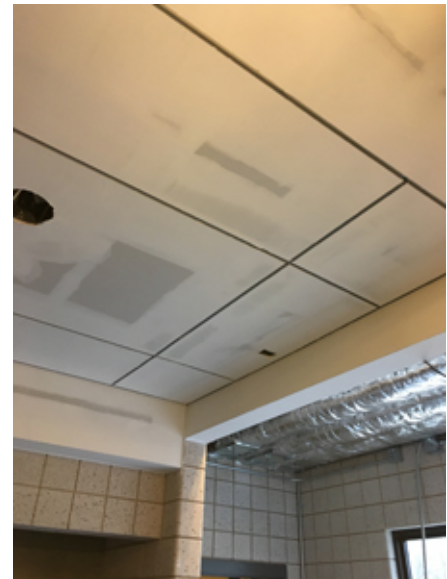
2018.11.26 – The reveals in the ceiling near the display case have been completed.
