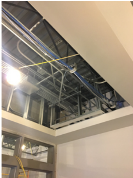
2018.11.19 – The bulkhead in the Office area has been constructed.
