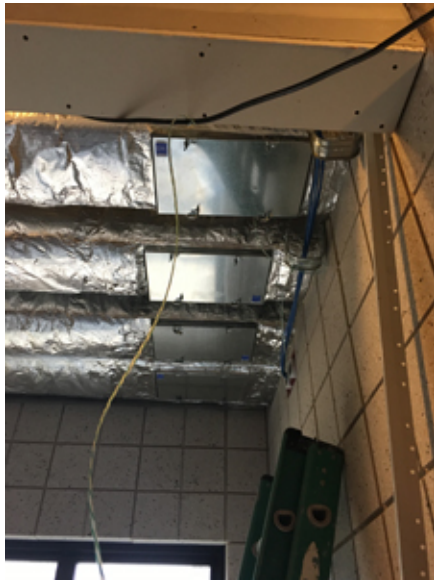
2018.11.19 – Access panels have been installed in the ductwork.
