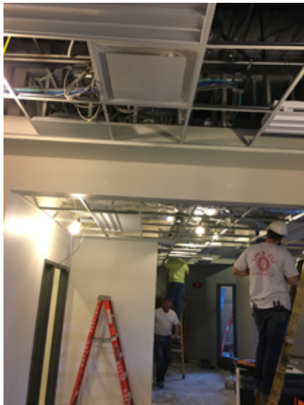
2018.11.26 – Installation of the ceiling grid, light fixtures, hvac grilles and diffusers has started.
