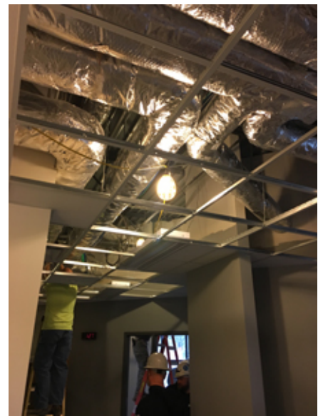
2018.11.26 – Installation of the ceiling grid is in progress in the office area.
