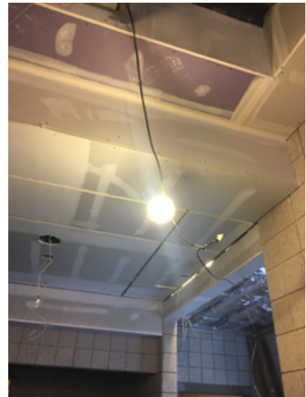
2018.11.19 – Installation of the reveals is in progress at the area of the display case.
