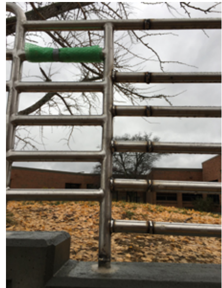
2018.11.26 – Finishing work on the stainless steel handrails is ongoing.
