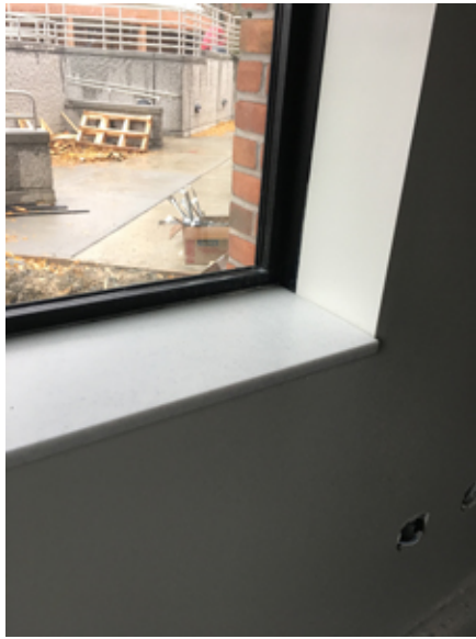
2018.11.26 – The solid surface window stools have been installed.
