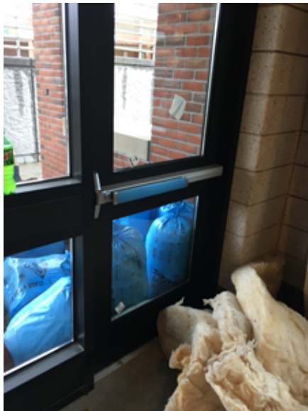
2018.11.26 – The doors have been hung on the main entry storefront system.
