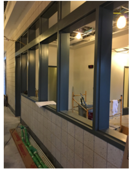
2018.11.26 – Final painting has started on the door and window frames.
