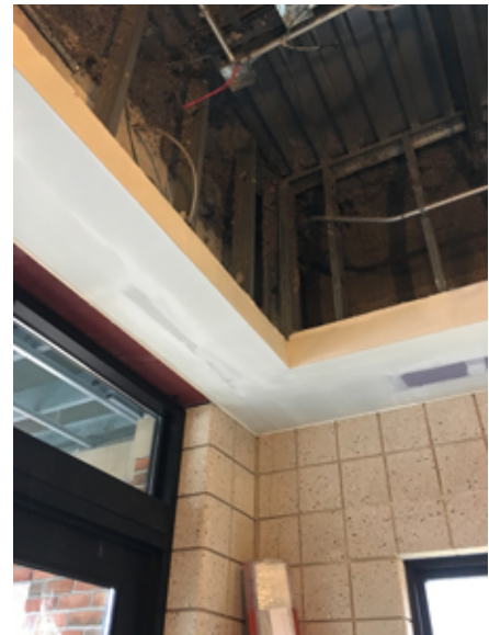
2018.11.26 – Finishing of the bulkhead in the Vestibule is in progress.
