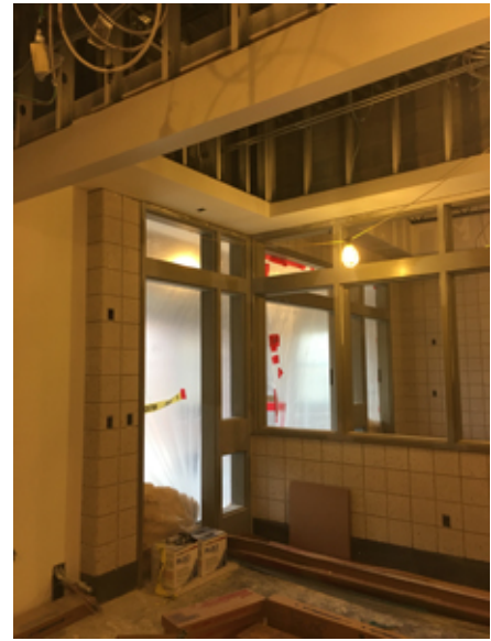
2018.11.19 – The bulkhead in the Office area has been constructed.
