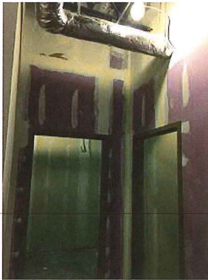
2018.11.05 – Finishing of the gypsum board continues.
