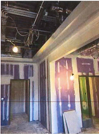
2018.11.05 – Finishing of the gypsum board continues.
