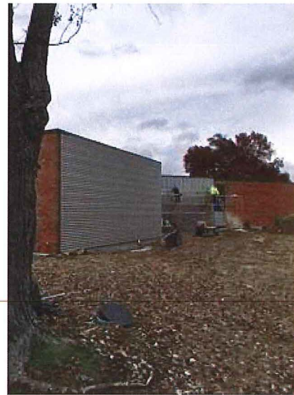
2018.11.05 – Installation of the metal siding continues.
