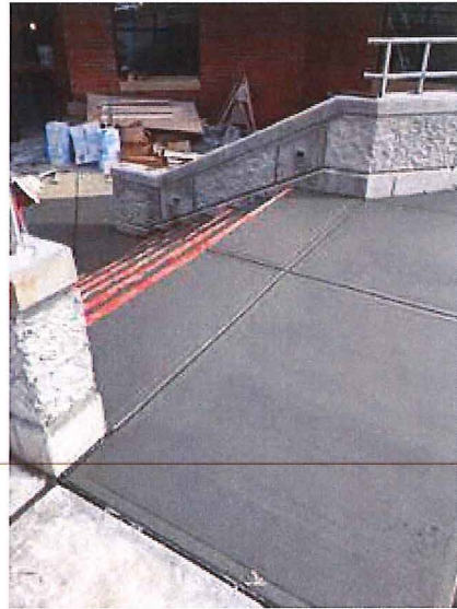
2018.11.05– The remaining concrete walk and stairs has been poured.
