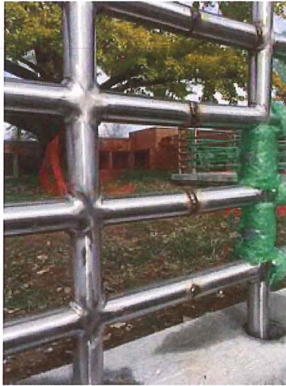
2018.11.05 – Repair of the stainless steel handrails is in progress.
