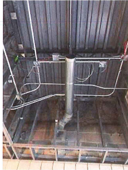
2018.10.31 – The joint between the metal roof deck and exterior walls has been insulated.
