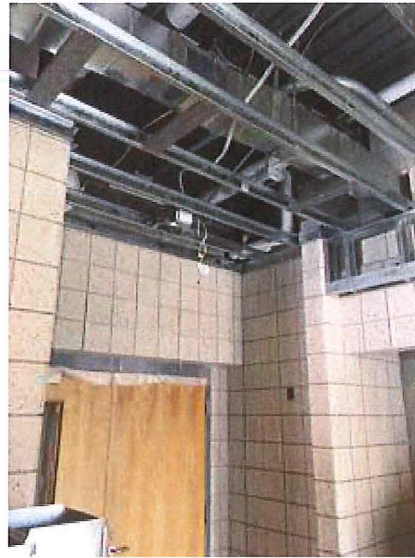
2018.10.31 – Installation of ceiling and bulkhead framing continues.
