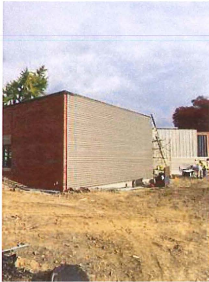
2018.10.31 – Installation of the metal siding has started on the rear of the building.
