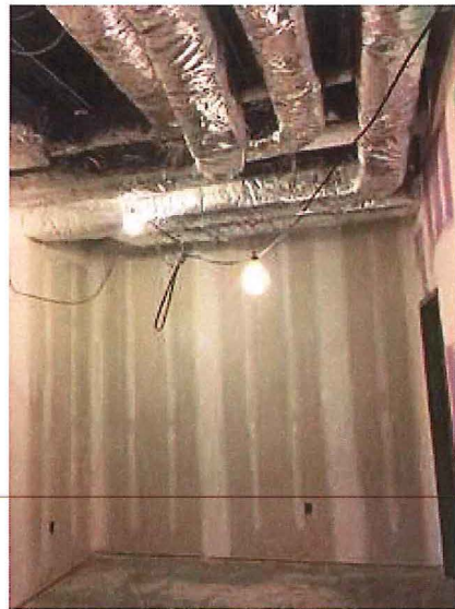
2018.11.11 – Finishing of the drywall continues. The Level 5 finish still needs to be completed.
