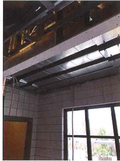
2018.11.05 – Installaton of the ductwork continues.
