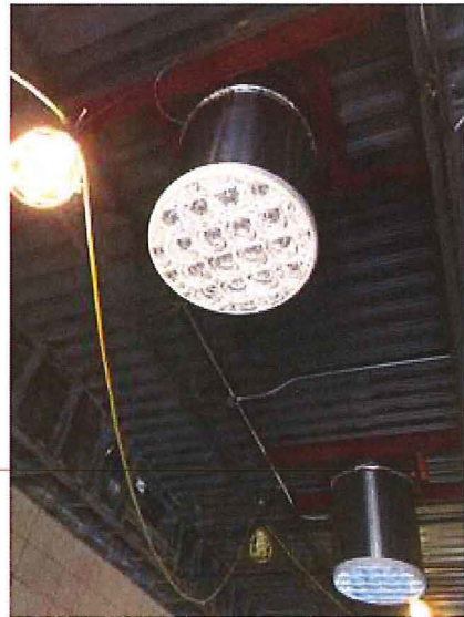
2018.10.31 – View of the solar tubes in the Lobby area
