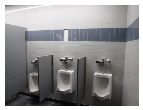
k) A significant number of wall tiles are not in plane with the rest of the wall. These must be replaced.
