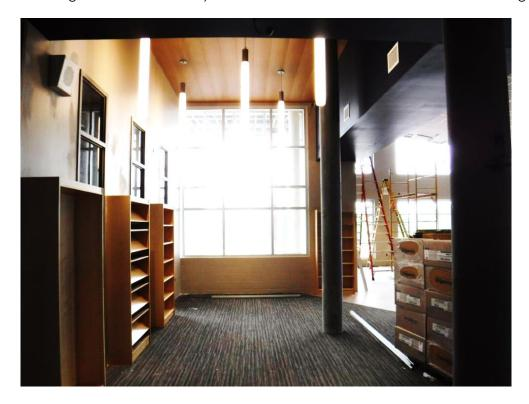
s) The gypsum board chase wall has been installed to cover the ductwork in the Library Office/ Storage Room.
