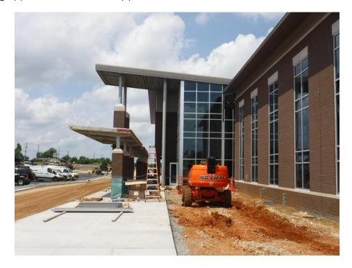
e) Mike Billings and I discussed the location and heights of the light bases for the building signage. The ground is not at the finished elevation. It will be flat at the base of the brick walls. JRA will issue instructions concerning the earth being placed over the through wall flashings.
