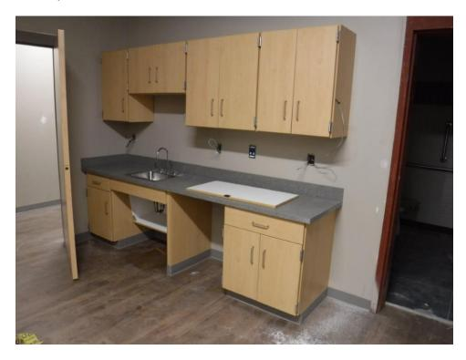
o) The casework and countertop in reception were installed. Coordinate the location of grommets cut into the countertop with HCS.
