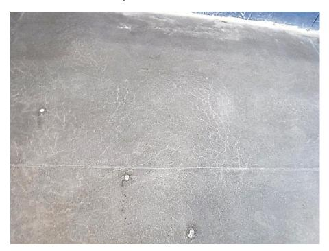
w) Some slab areas have had significant damage. With the contrasting repair, these areas are emphasized.
