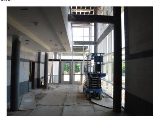
o) Conley Painting used balloons to mask the can lights as they sprayed painted the ceilings and soffits over the main corridor.
