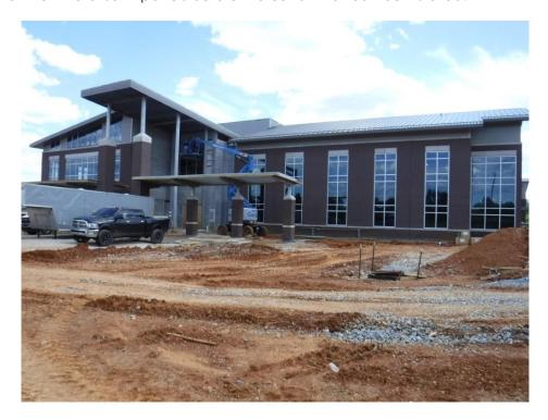
c) Now that Dixie Exteriors is back on site from a standdown due to a COVID – 19 outbreak in their crew, they are completing the installation of the fiber cement panels under the roof soffits on the classroom wings.
