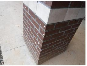
u) Brick had been removed to correct the distorted door frame into the Band Room.
