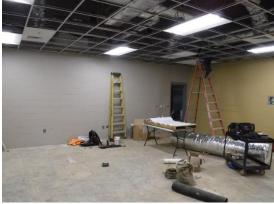
j) The edge trim for the ceiling clouds has arrived on site. Ceiling installers were assembling the clouds on the floors of the rooms prior to lifting them into place.
