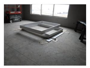
k) Work continues for the installation of gypsum board soffits. These along with the walls will define the edge for lay in ceilings.
