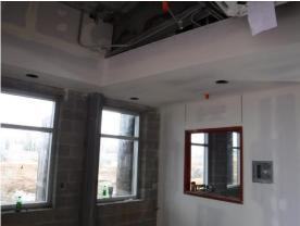
l) Light gauge metal framing was being installed along the walls on the second floor of the main corridor.
