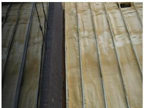
e) Spray foam insulation was not applied in the corner between the last "Z" and the brick returns at the cafeteria. This is also the case on the other side of this wall where the expansion joint is to be installed as noted above.
