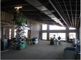
y) Glazers were installing insulating glass units in the ends of the classroom wings.
