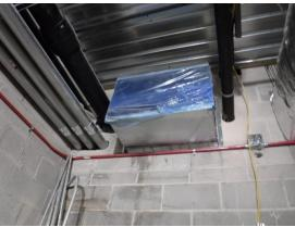
d) Doyle confirmed that the electrical conduits pasting through the two-hour fire resistive rated fire walls would be sealed with fire resistive sealant. The sealant must be installed based on a U/L fire resistant rated assembly for the spacing and size of the conduits.
