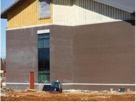
z) Glass has been installed at the exterior of the Library/Media Center except for those at the top which need the composite panels before the window installation.
