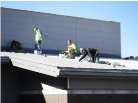
o) The roof over Area D in front of the gym was covered with mud and debris from the spray foam and panel installation process. We discussed the need to prevent this from happening again. Workers will change shoes when moving from the ground to roof areas and materials will be cleaned before they are raised to the roof.
