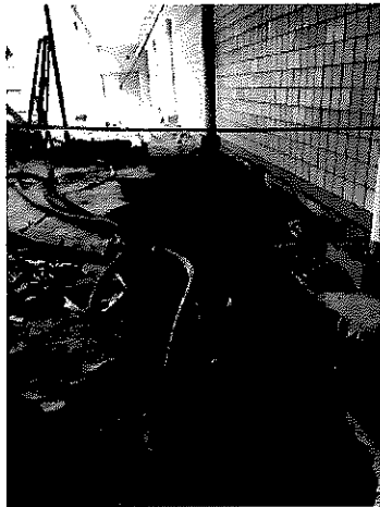
2018.07.03 – Backfilled sanitary trench along fire wall.
