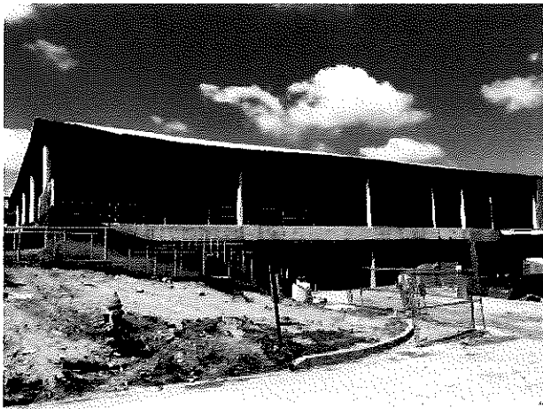
2018.06.28 – Exterior skin removed at East elevation.
