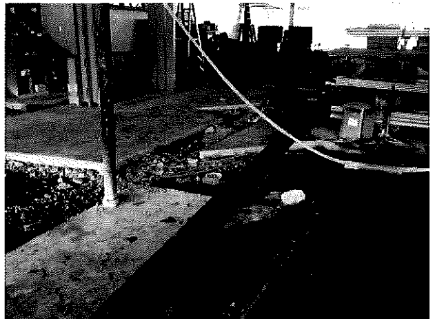
2018.06.28 – Geothermal piping to be pulled back through the bored hole.
