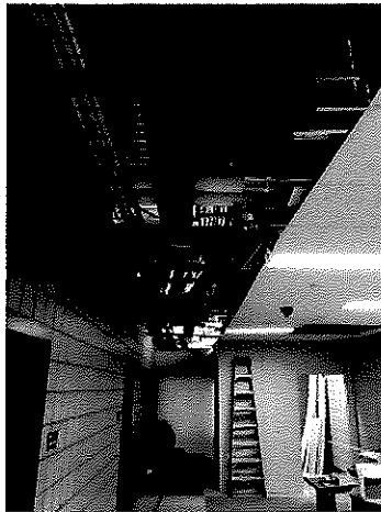
2018.07.17 – Buss duct above Phase 2B ceiling.
