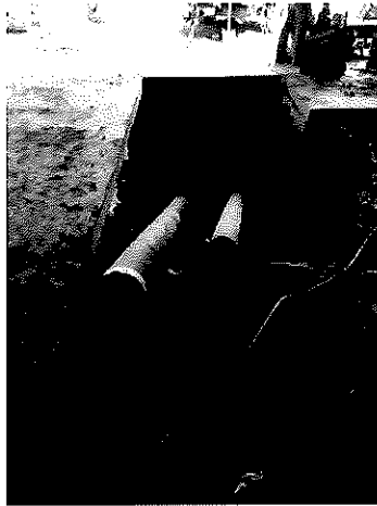
2018.07.03 – Geothermal laterals visible inside the building.
