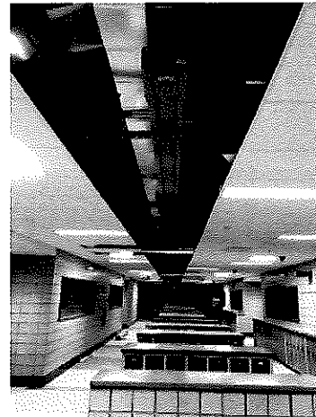
2018.07.17 – Buss duct above Phase 2B ceiling.
